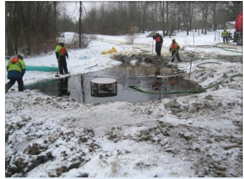
Vacuuming of raw product at Peck Wadsworth Road dam (Courtesy of Wellington Fire Dept.)
