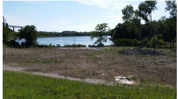
ODNR Rookery Restoration Project Immediately After Construction: Courtesy of Coldwater Consulting
